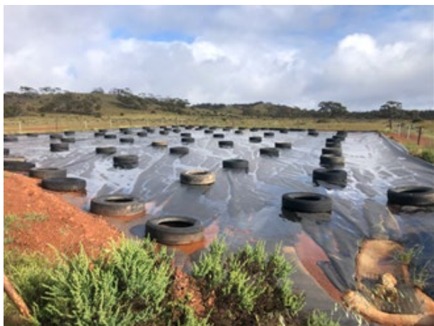
Lined catchment immediately above dam
