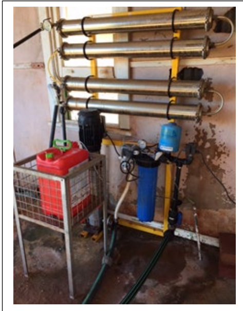
Puredrop 4 membrane desalination plant on Mt Eba
