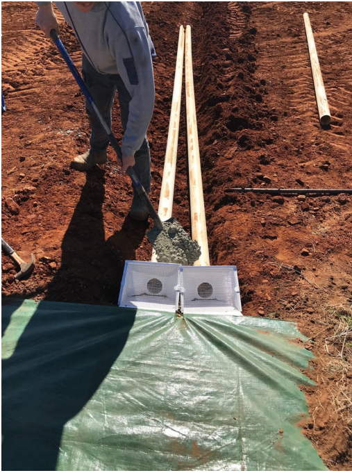
Installing the sump
