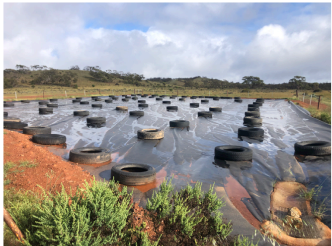
The lined catchment situated immediately above an existing dam on Dale's property
