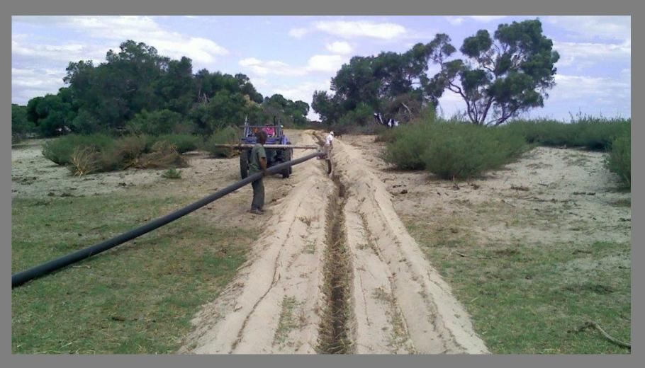
Piping water from Lake Albert or from a bore with fit for purpose water Can be 15kms +
